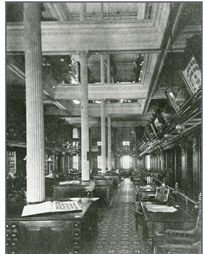
A view of the new State Library from the second floor, circa 1879. Corinthian cast iron columns supported iron beams that ran through the open center of the room at the third and fourth floor levels. These beams supported the weight of the balconies and bookshelves bordering the room on the upper floors.
