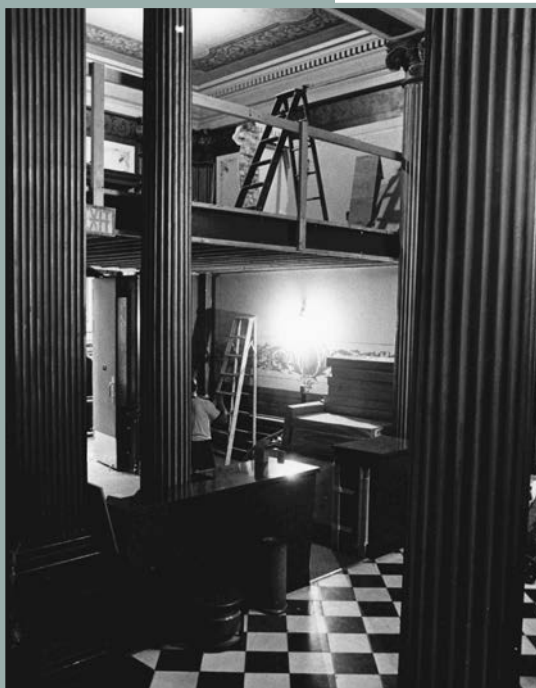
Offices, corridors, and even the lobby into the House Chamber, seen here, were sliced in half horizontally to create additional office space in the late 1960s and early 1970s.
