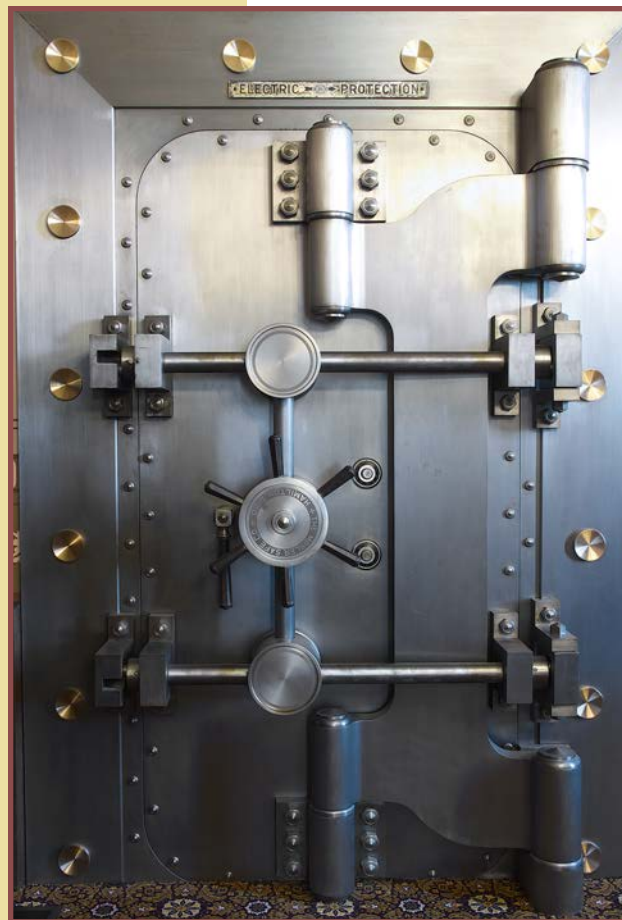
The sleek, streamlined 1924 Mosler vault door is both a symbol of governmental strength and an object of beauty from the Art Deco era.
